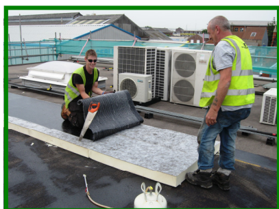
Office Roof Insulation
